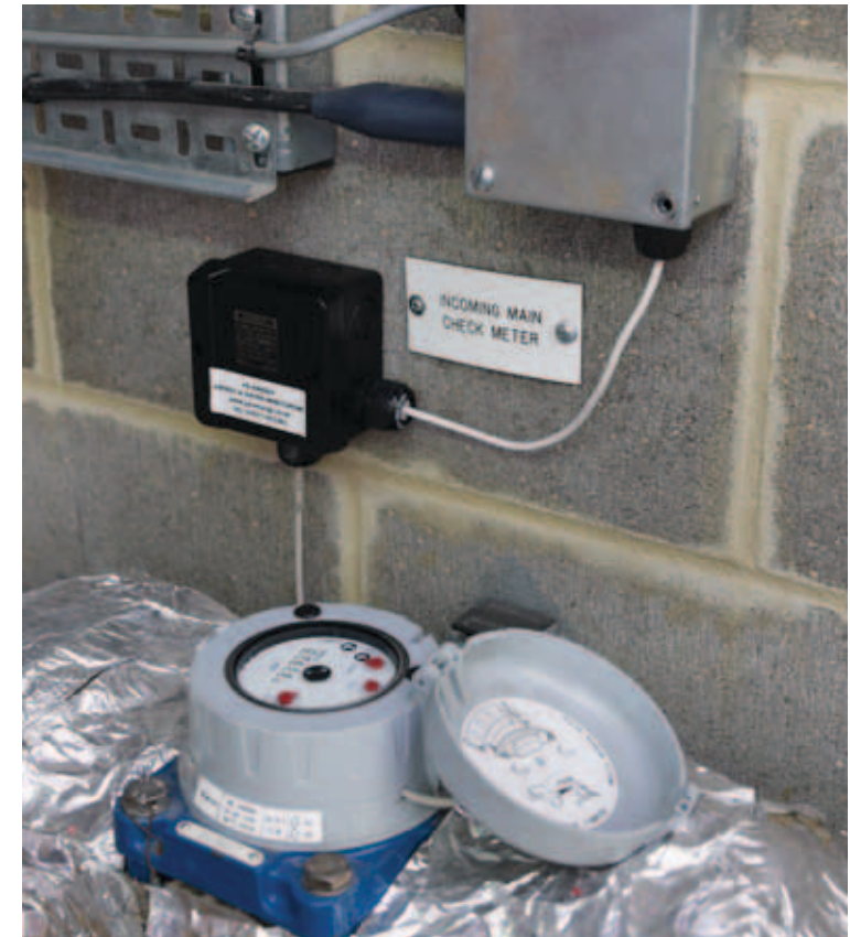
Figure 18: Hard wired cabling installation for internal transmission of main water meter pulses
