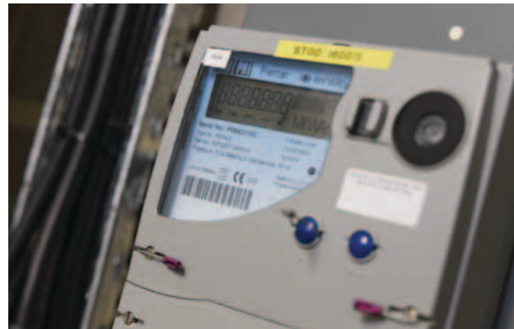
Figure 10: Main electricity meter
