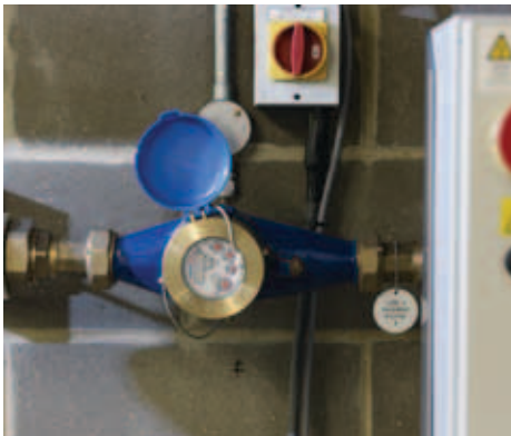
Figure 14: AMR capable water sub-meter
