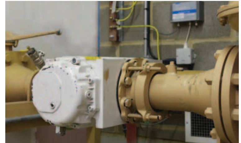
Figure 12: Main gas meter
