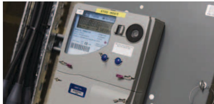
Figure 4: Main electricity meter
