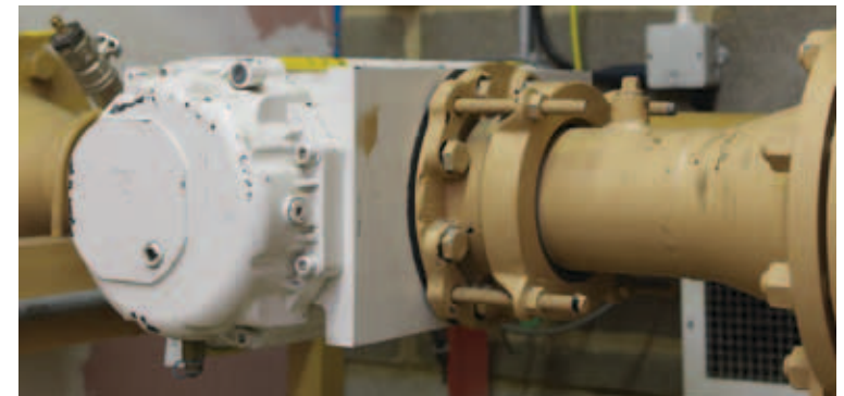
Figure 5: Main gas meter
