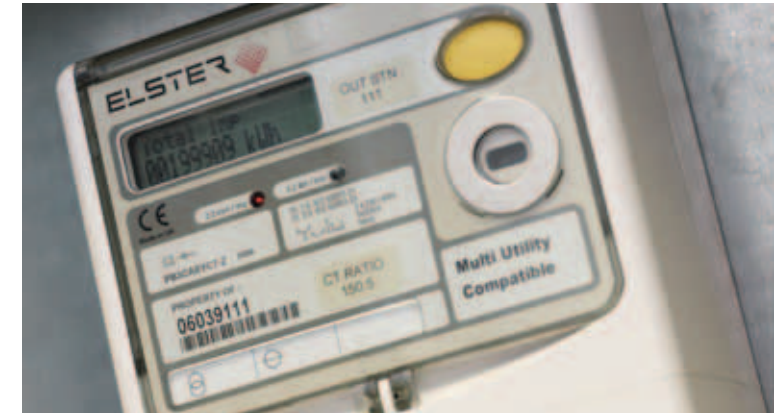
Figure 15: Electricity sub-metering of a photovoltaic array
