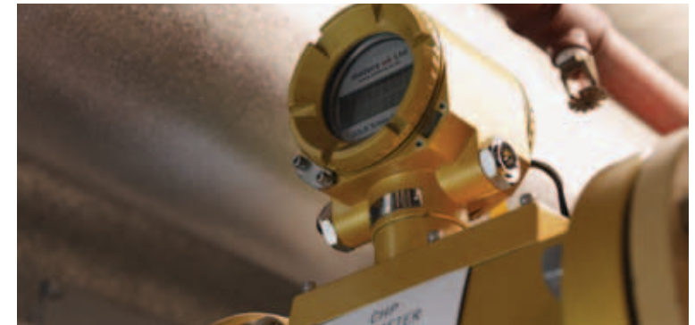
Figure 8: Gas sub-meter for a Combined Heat and Power (CHP) engine
