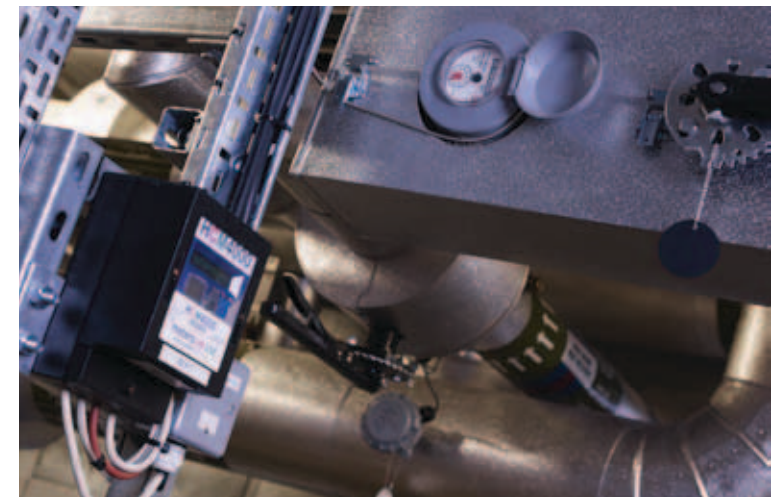
Figure 9: Heat and coolth sub-meter
