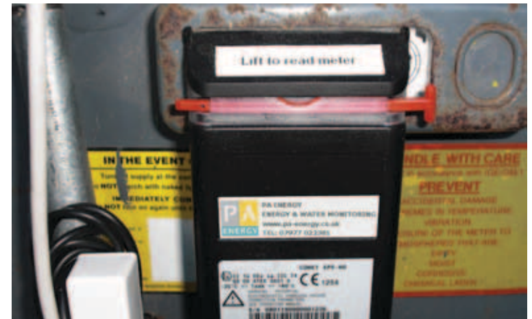
Figure 13: Optical reader (courtesy of PA Energy)
