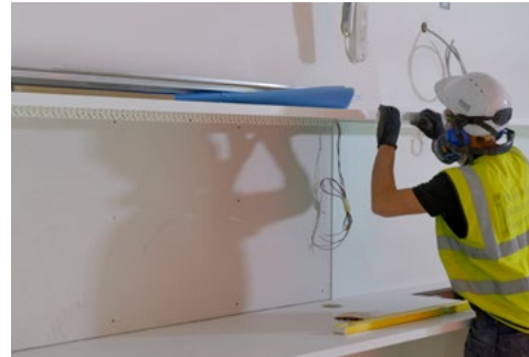
Fitting out apartments at Rathbone Square, W1
