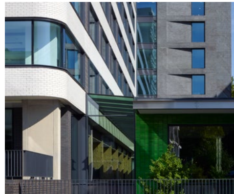
The new podium floor at 160 Old Street, EC1
