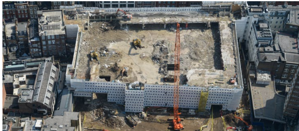
The demolition phase at Rathbone Square, W1
