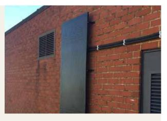
At Crosspoint House, Wallington, Surrey and in conjunction with Magic Box International, CLS has completed its first installation of a thermodynamic hot water system . This innovative technology uses a special solar panel combined with a heat pump to meet all of the hot water needs of the building. The system provides cheaper hot water to our tenants, increases our use of renewable energy and reduces the impact our buildings have on the environment.
